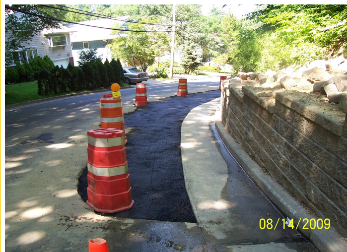
Picture 8—A base layer of asphalt is laid.
