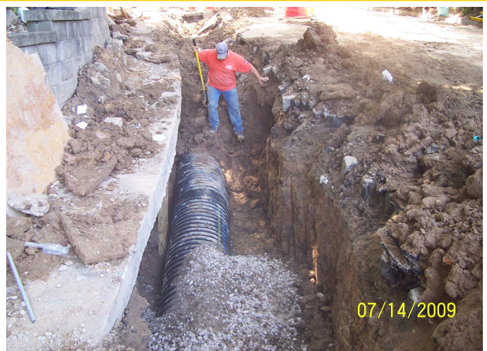
Picture 5—a new section of storm water pipe is laid and backfilled by Dave Distili.
