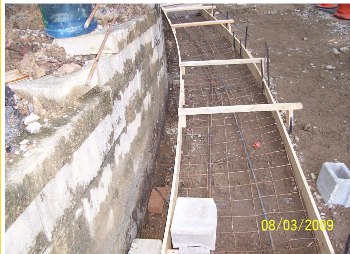
Picture 6—Framing for the concrete curb and shoulder is laid out.
