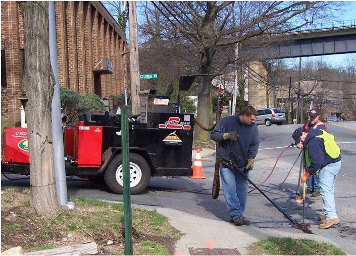
DPW crew crack sealing, an integral part of the Village's road maintenance plan.
