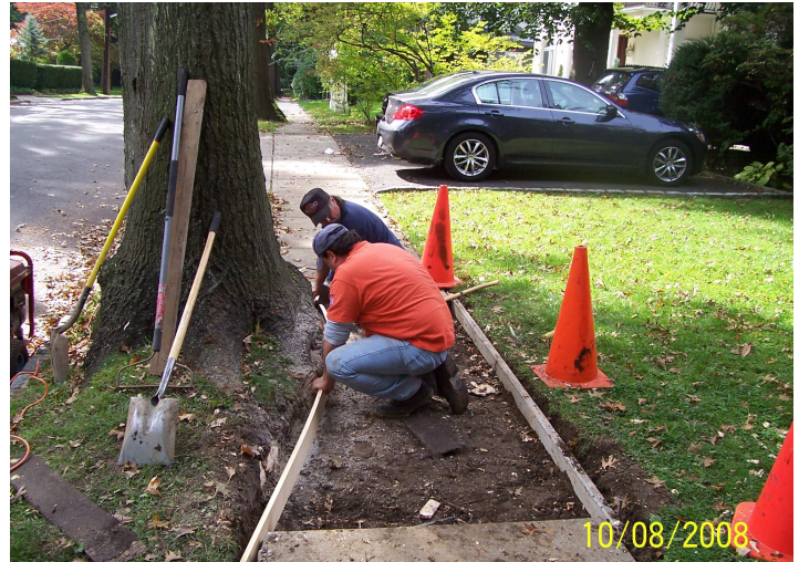
DPW crew repairing a sidewalk in the Village. Recently, Supt. Mazurkiewicz began using a new technique when pouring cement which is designed to prevent sidewalk sections from lifting unevenly and creating a trip hazard.
